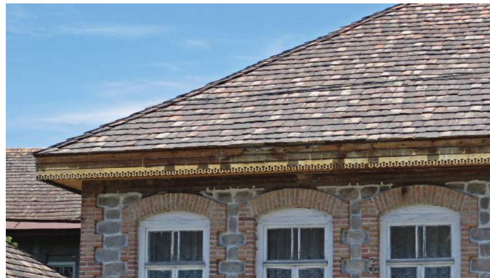
FIGURE 106: Typical wooden cornices hand-carved according to traditional patterns
