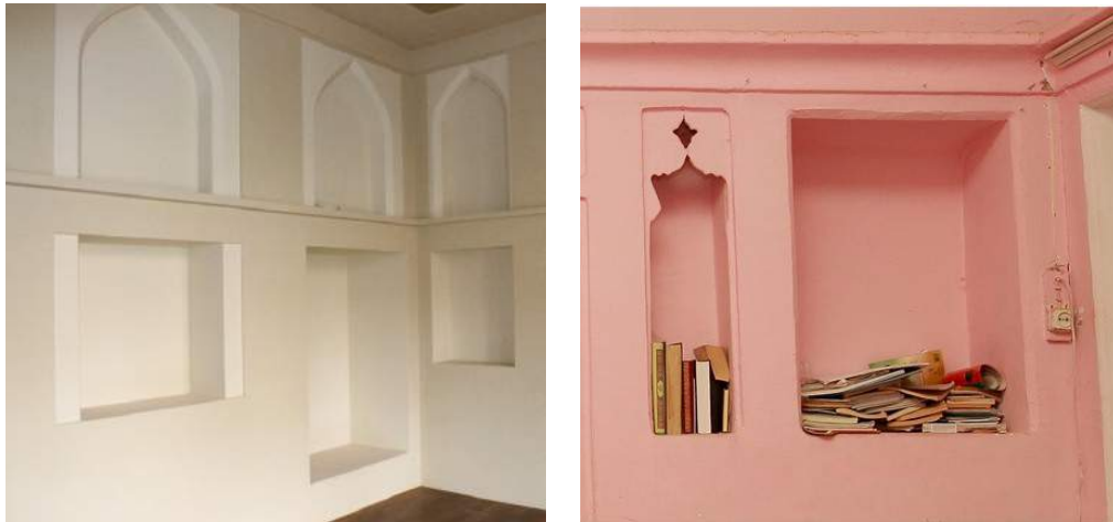
FIGURE 87: The traditional houses have many wall niches serving storage functionals but also used to lighten the walls and create sub-rigid structures with anti-seismic function. They are mostly found on the upper floors
