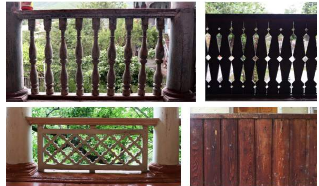
FIGURE 104: Wooden balustrades are divided into four groups according to manufacturing techniques: a) with balusters carved of wood; b) with flat balusters cut from wood; c) with fretwork instead of balusters; and d) with wooden panels.
