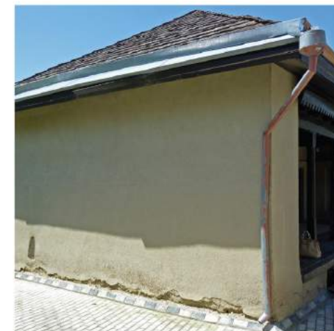
FIGURE 137: Simple or decorated in the traditional style, the gutters and the downspouts are necessary to reduce the rapid deterioration of the overhanging structures and of the underlying walls due to uncontrolled waters. The colour must be copper or weathering steel, or a pre-rusted material should be used. This colour is integrated with the roof tiles. The pipes are often decorated. This is a recent tradition that should be perpetuated and incentivized.
