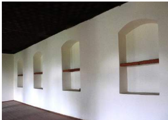
FIGURE 88: Some large niches are divided into several horizontal compartments with wooden shelves.
