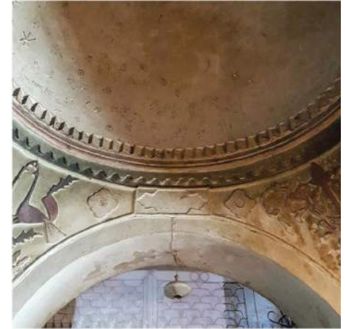
FIGURE 100: Ornaments are subject to various degradation factors such as chromatic alterations, cracks and fractures, and surface contamination. Moreover, they are frequently contaminated with elements, forms, and materials outside the historical context.
