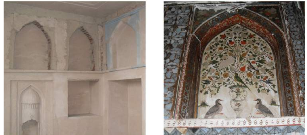
FIGURE 89: Arches and niches are subject to fractures. Other degradation factors include the accumulation of foreign bodies in decorative parts, and the formation of cavities, as well as incongruous additions.
