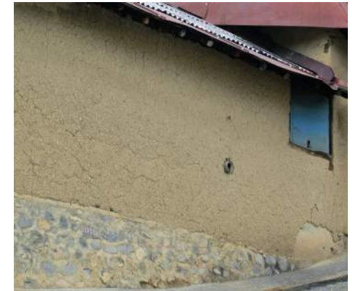
FIGURE 129: Buildings with mud wall, the outer surface is smoothed first with mud and then plastered with clay. This technique improves the resistance of masonry to the erosion.
