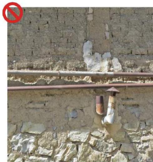
FIGURE 135: The side vent should only be installed in the inner courtyard and never on the main street and respect the colour of the wall on which it is placed (e.g. shades of grey are admissible on stone).
