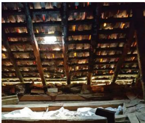
FIGURE 59: The chimney pot visible in the attic, lit by soft light filtering between the tiles and the skylight.
