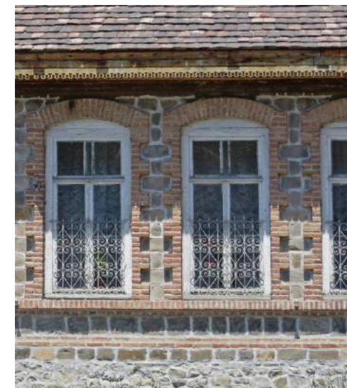
FIGURE 71: Traditional windows with wrought iron railings
