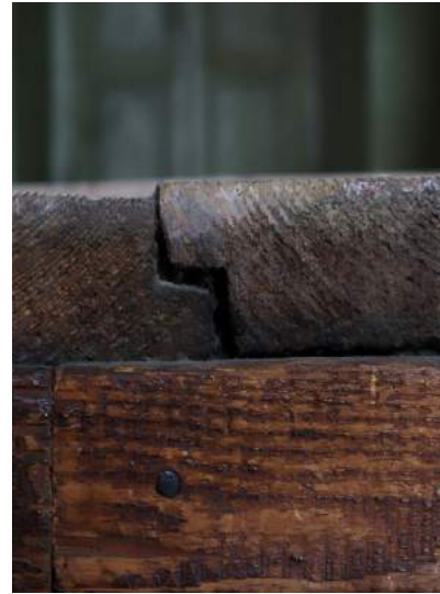
Figure 32: Technique for joining floorboards
