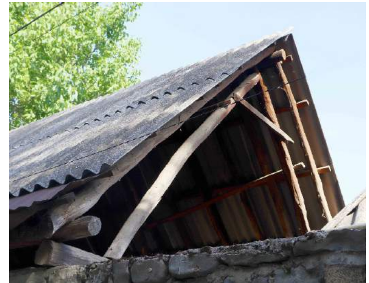
FIGURE 25: Scissors truss
