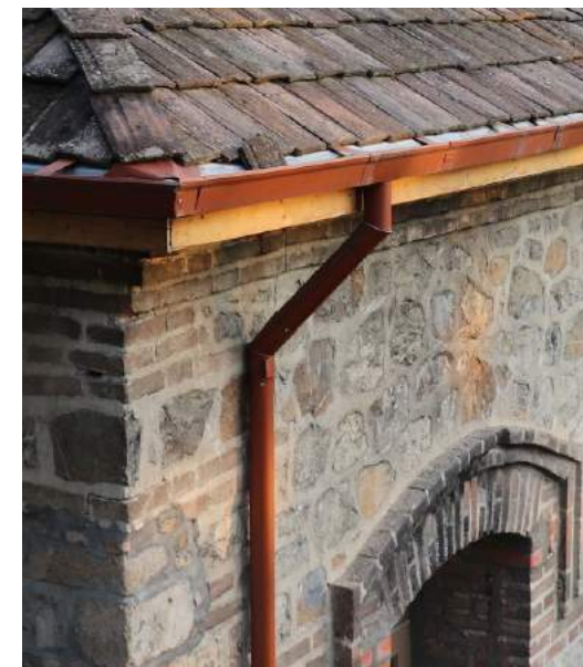
FIGURE 61: Correct roof drainage system
