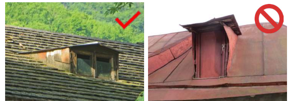
FIGURE 57: Dormer windows must be in compact and small forms that follow the historical style dictated by the Khan's Palace. Maximum two windows can be installed respecting the symmetry and not facing the main road.
