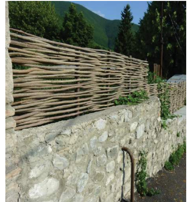
FIGURE 93: Newly restored boundary walls in Sheki Fortress
