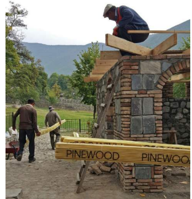
FIGURE 118: Pinewood is a type of coniferous wood suitable for the use of roof structures, for its resistance to xylophage agents.
