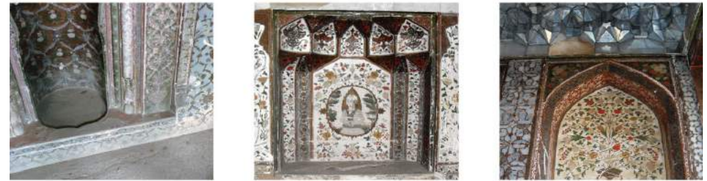
FIGURE 116: Deterioration of frescoes and loss of original colours
