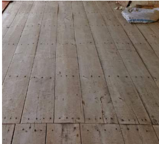
FIGURE 119: Re-use of some well-preserved old wooden planks
