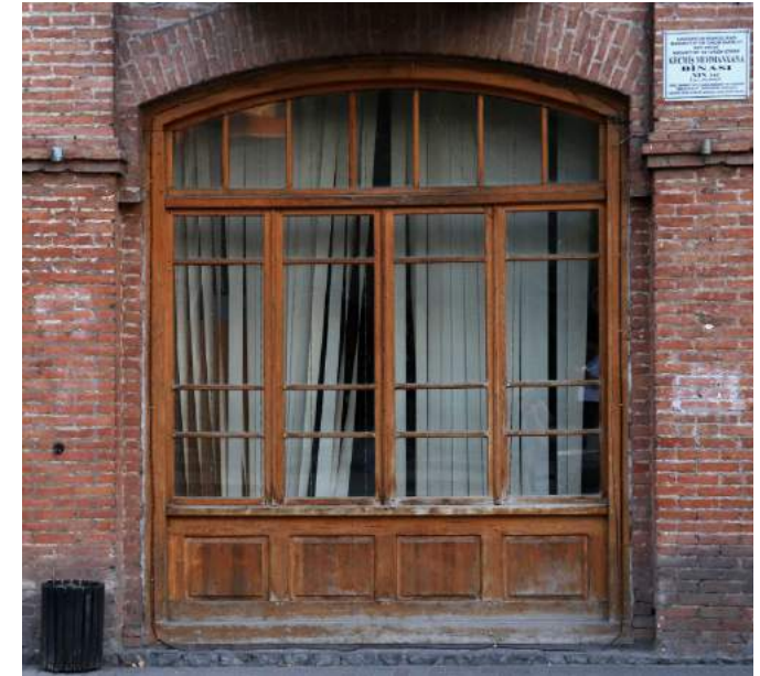
FIGURE 74: Preserved window on the ground floor of a public building
