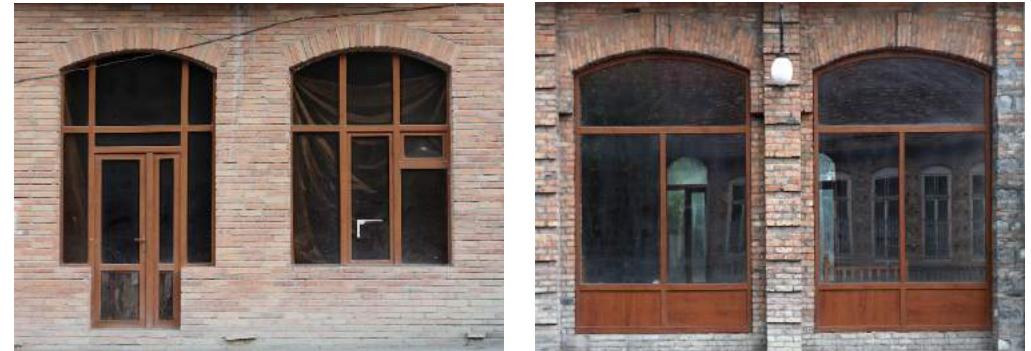
FIGURE 75: Two examples of PVC casings. The casing on the left is more reminiscent of old wooden frames but the casing on the right is rather simple and incongruous.
