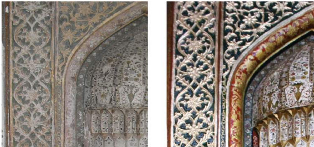
FIGURE 102: Cleaning the ornaments with the absorbent wrapping technique which involves the use of substances with high absorbency capacity such as cellulose pulp, carboxymethyl cellulose, talc, colloidal silica and some particular types of clays (bentonite, meerschaum, and attapulgitite).
