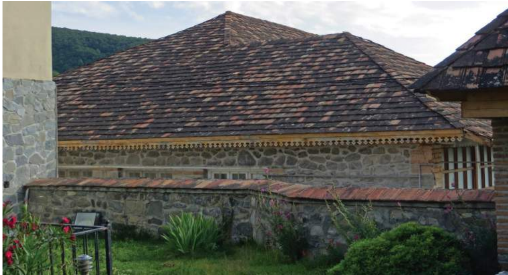
FIGURE 91: Traditional walls made of river stones using limestone mortar
