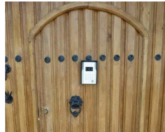
FIGURE 138: Bad example of an intercom on an old door.
