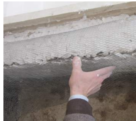
FIGURE 101: Metal mesh should be placed between the mortar and the substrate to make the reconstructed decorative elements durable.
