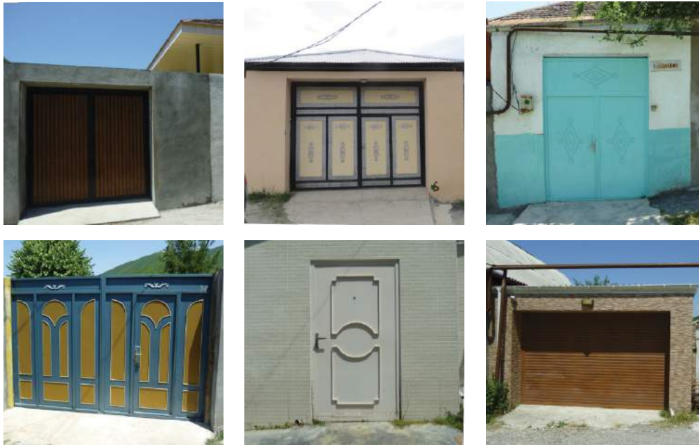
FIGURE 66: Modern gates and doors that contradict the traditional gate typology of Sheki in terms of shape and material use
