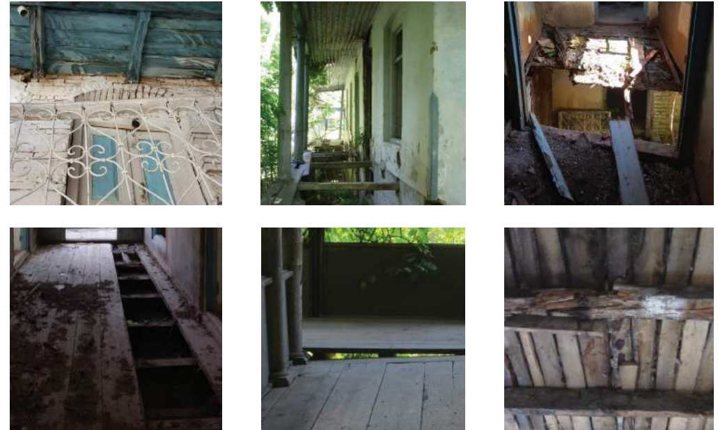
FIGURE 34: Moisture is one of the main causes of wood degradation. Causes of moisture include capillarity – the movement of water through the pores, hygroscopic effect – the absorption of moisture in the air, condensation of atmospheric humidity and infiltration factors.
