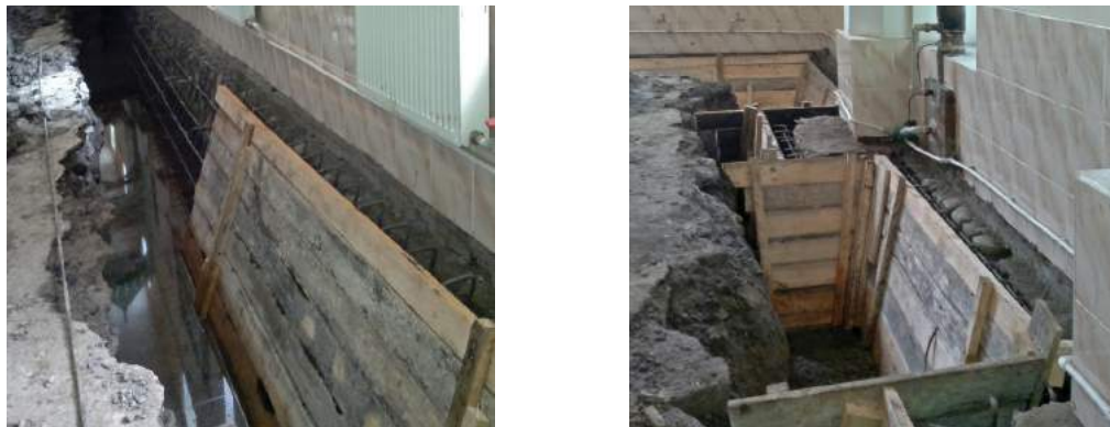
FIGURE 14: Rehabilitation of the foundation by reinforcing work with concrete beams
