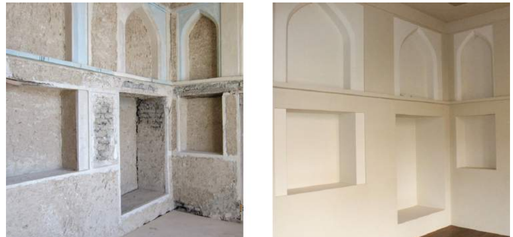
FIGURE 90: Correctly restored wall niches
