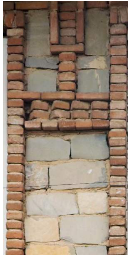
FIGURE 123: Sorted river stones were carved in a rectangular shape and mostly used in combination with fired bricks.
