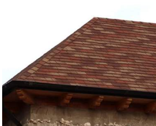
FIGURE 58: From modern materials, only soft materials that look like traditional tiles are allowed
