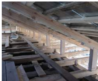
FIGURE 29: Replacement of damaged parts of the truss
