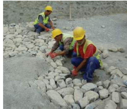
FIGURE 122: Due to their rounded surface, river stones are mostly used for paving the streets.
