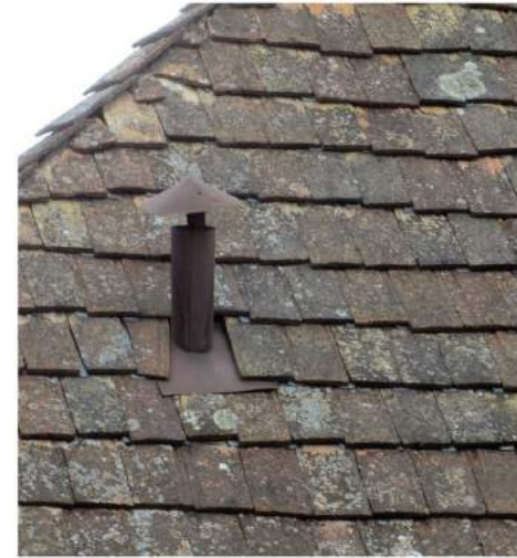
FIGURE 134: Possible installation of chimneys must consider the context and be non-invasive, fitting with the colours of the roof for a less visual impact.
